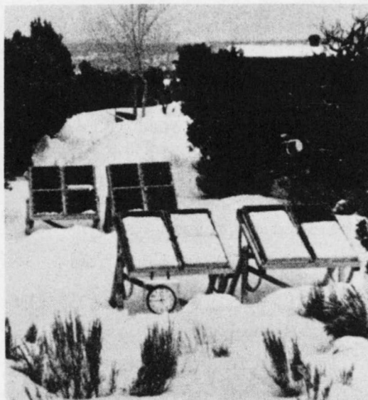
11:45: 40° PANELS ARE CLEAR, 30° PANELS ARE BEGINNING TO SHED.
